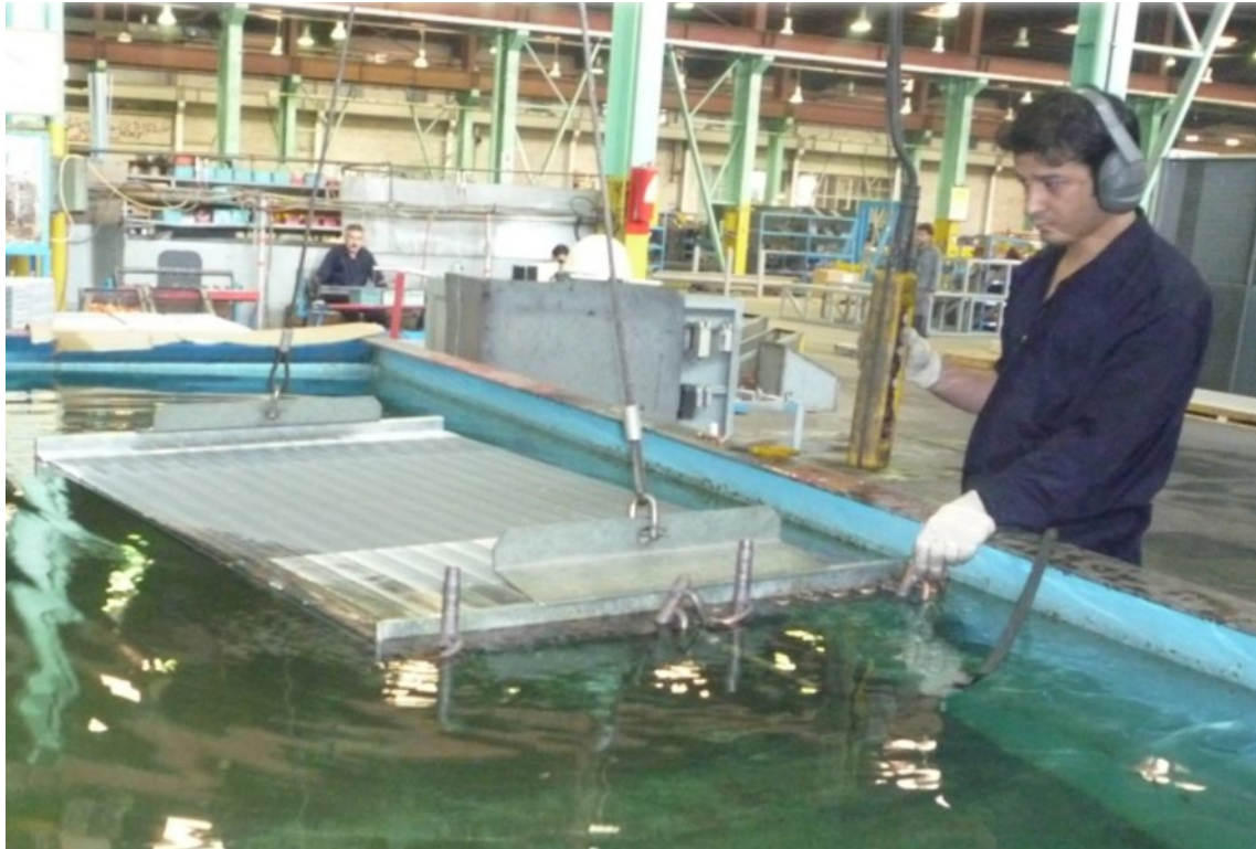
Pressure Test of Heat Exchangers
